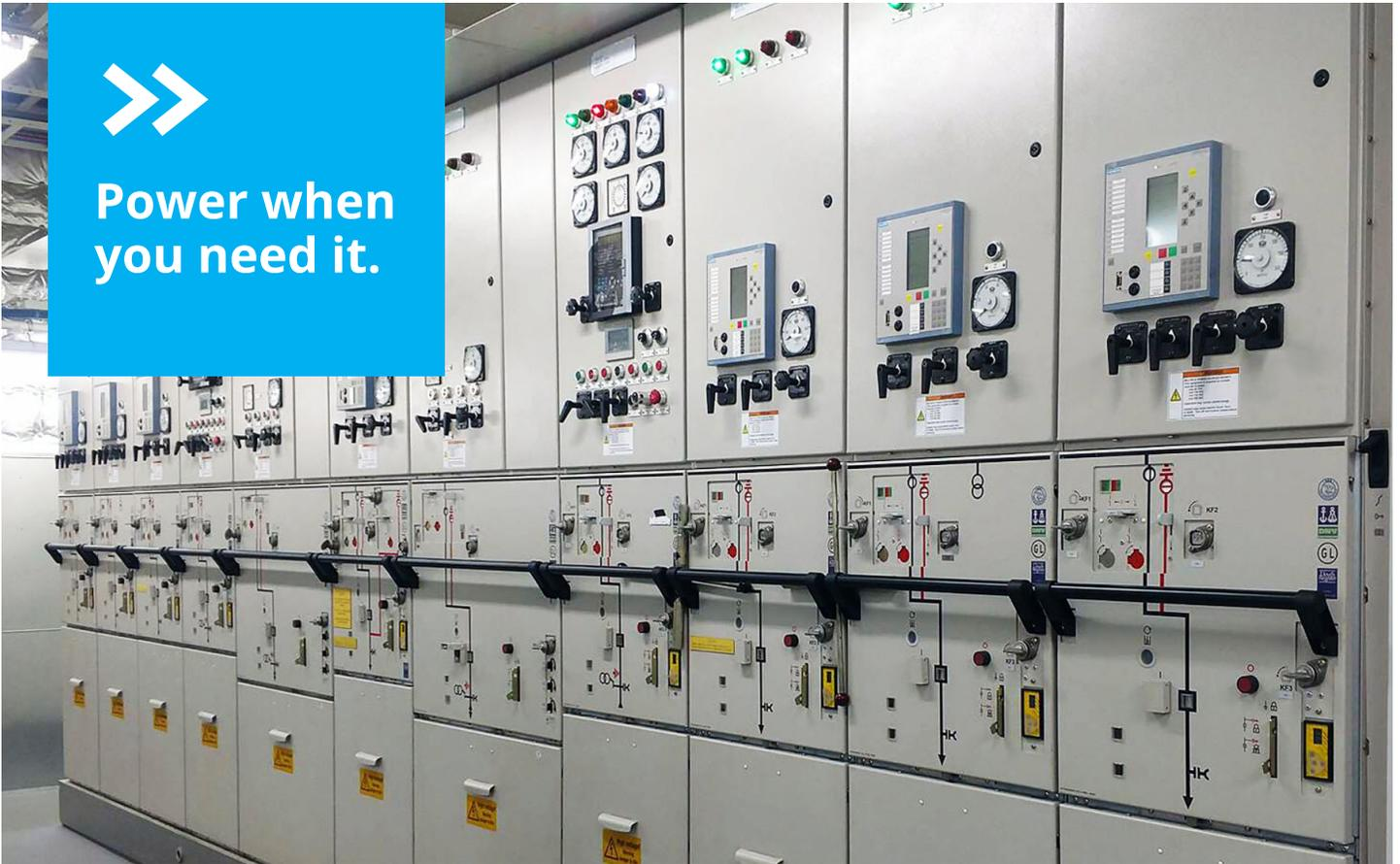
The AGP system coordinates multiple sub-systems in a unique architecture that is founded on fault tolerance. By monitoring the various generator incomers, tie breakers, and overall power distribution, the AGP can predict vessel events to prevent or minimize their effects.
