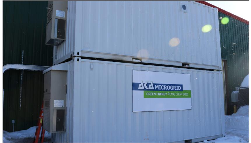
AKA's Pooles Corner Microgrid is designed focusing on power system reliability, power distribution management, and energy storage to support the campus including two facilities; manufacturing and AKA's START CENTRE: engineering building. It incorporates a diesel generator, renewable energy, and energy storage
